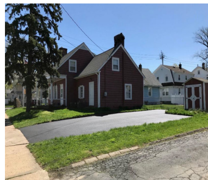
The Abraham Clark House with new driveway, roof, gutters, exterior painting and landscaping
